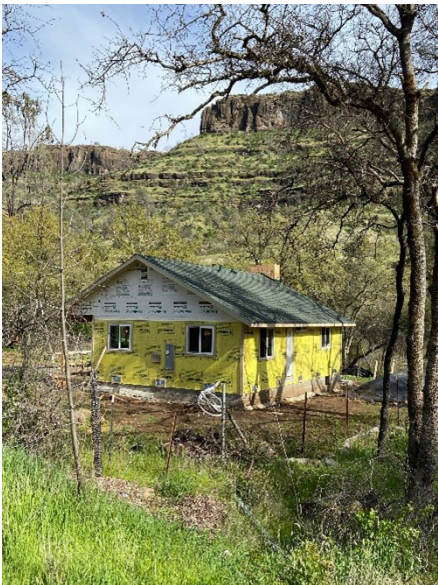
Figure 3: HRCB Caretaker Home Re-built by Students and Local Contractors
