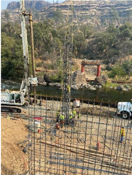
Figure 2: Pier 2 Construction with Abutment 1 in foreground
