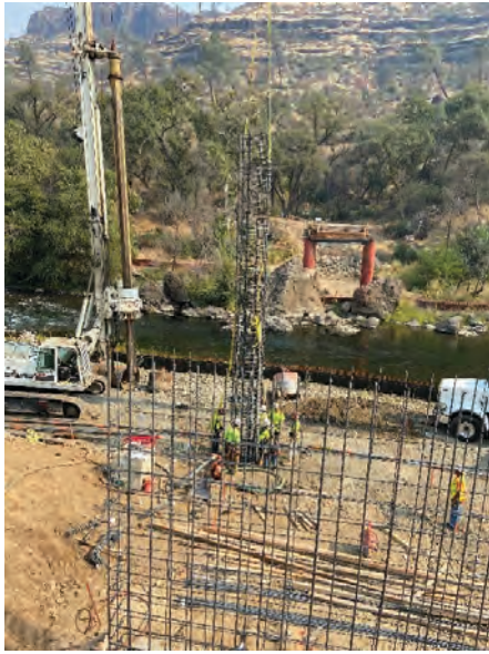
Figure 2: Pier 2 Construction with Abutment 1 in foreground
