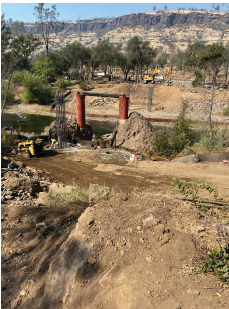
Figure 1: Pier 3 Construction Looking back at Abutment 1
