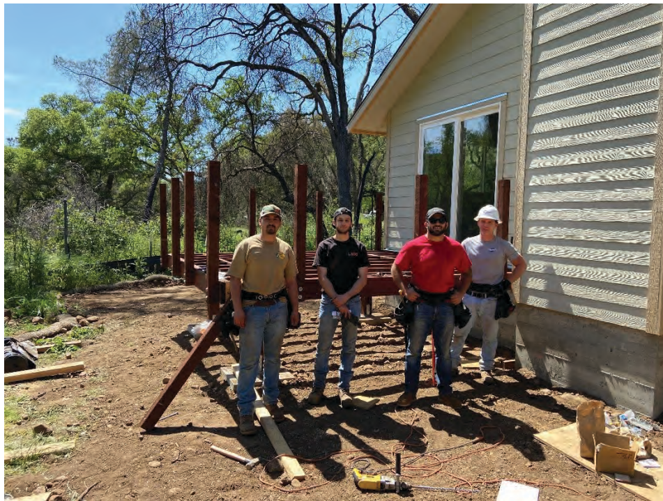
Figure 4: Chico State CMGT Students Finishing the Caretaker Home
